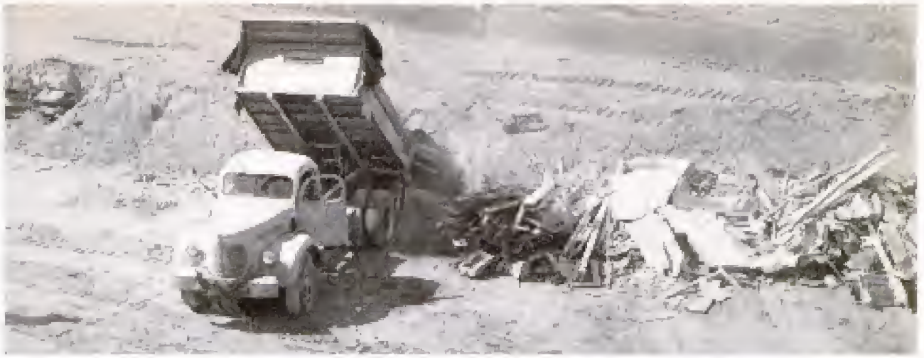
Truck dumps remains of radioactive building in 600-foot-long "grave" a safe distance from the laboratory
